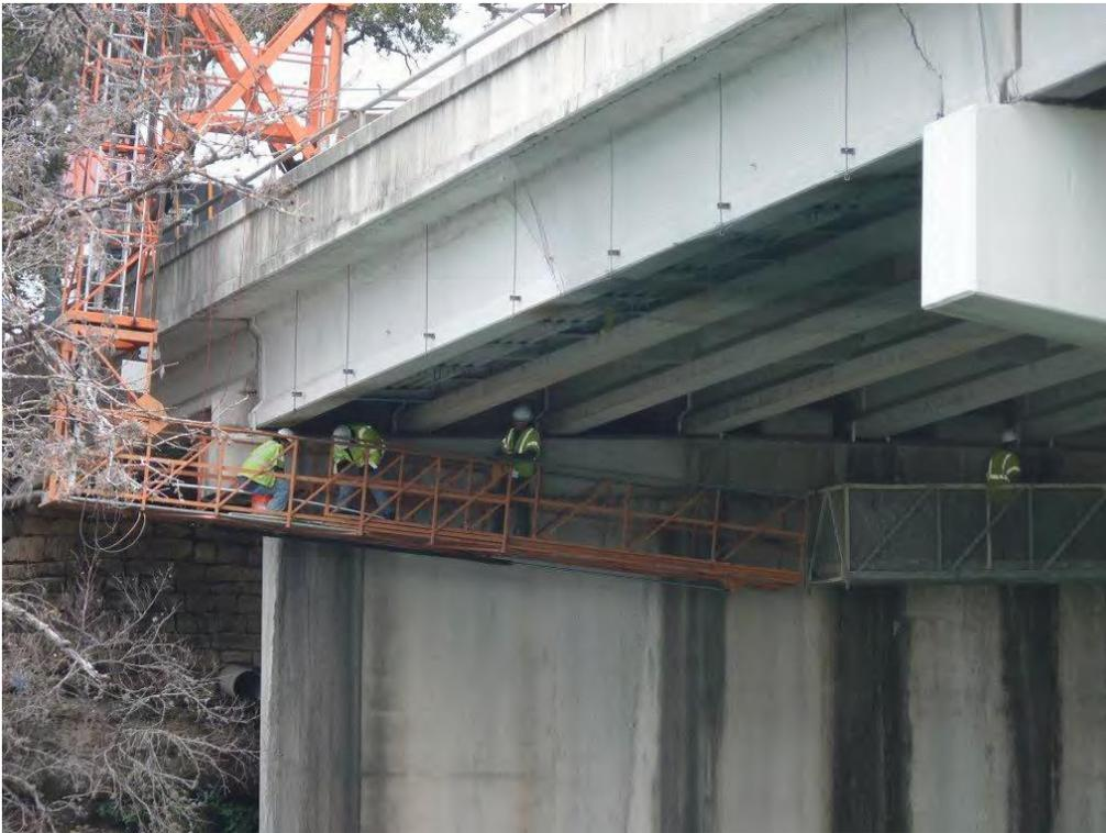
**Figure 13. Netting installation taking place on span of Hwy 16 Bridge over Guadalupe River**
